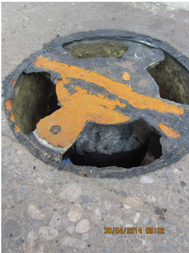
Detail Flutungsventile in Beckensohle
